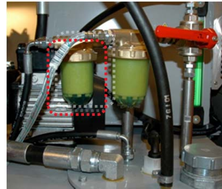
Aggregatets dieselfilter
